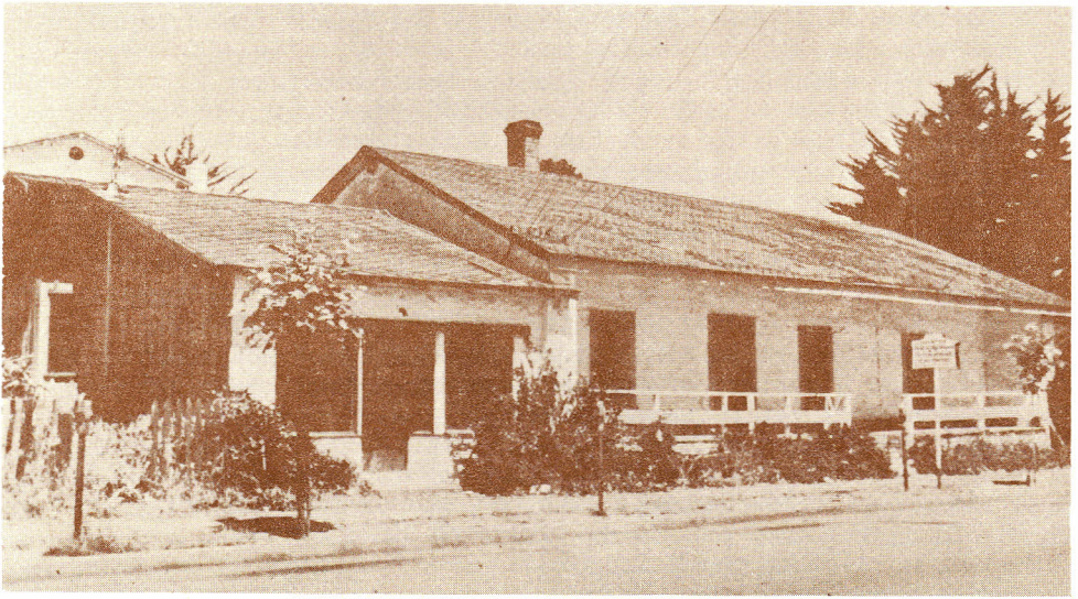
The Casa Serrano before the work of restoration had begun. Abandoned for years, the roof leaking, infested with rats, the rear buildings a hodge-podge of wooden board-and-bat additions, it was doomed to be razed by the bull-dozers.
