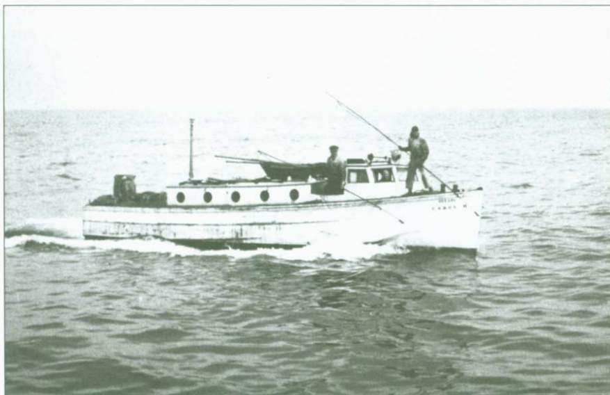
A basking shark boat similar to the Two Brothers. Note harpoons, rigging, and flotation barrels in stern. J.B. Phillips photograph, MHAA Collection.
