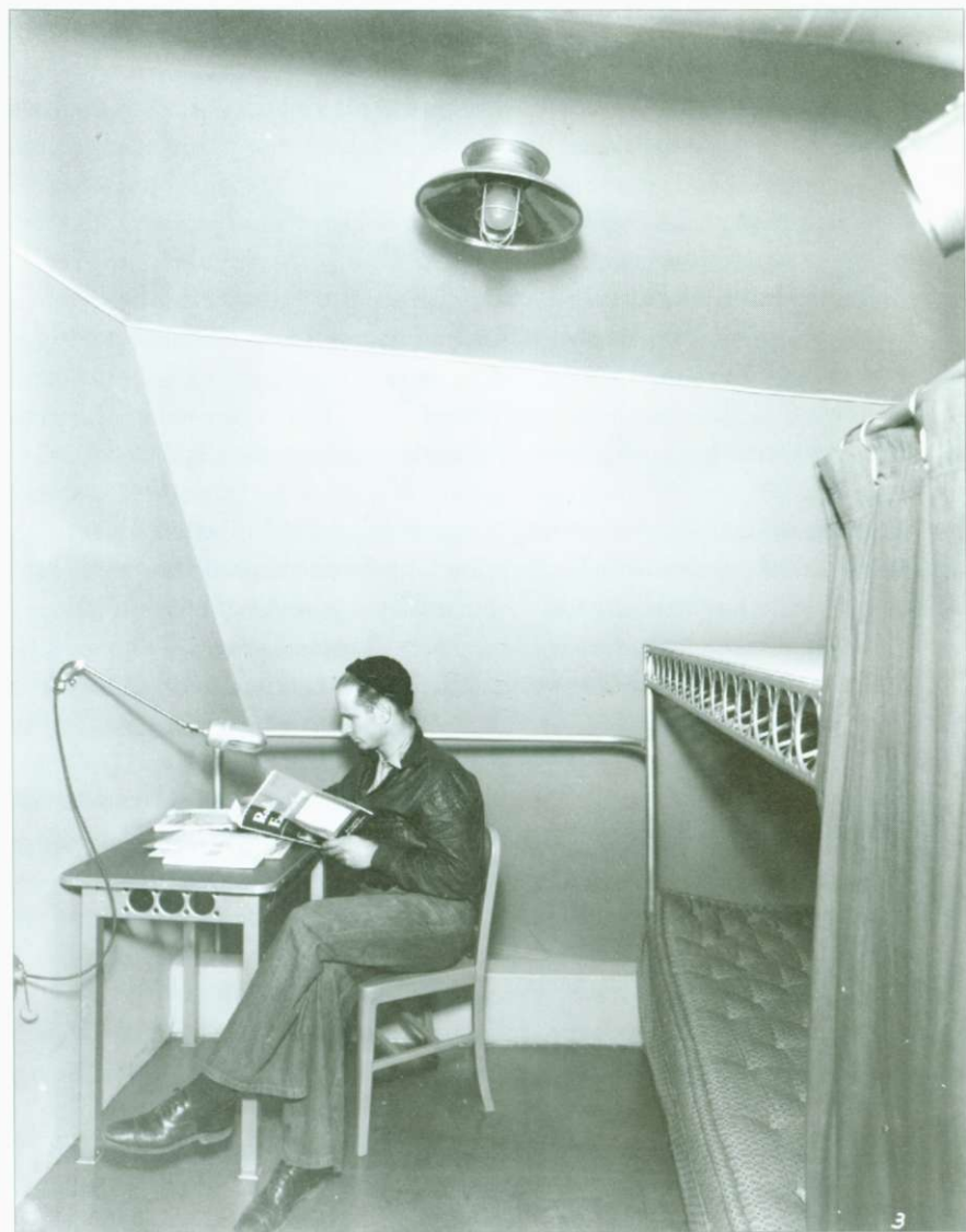
Interior of a cabin on the USS Macon; note the use of duraluminium girders on both desk and bunk bed. HVW photograph.
